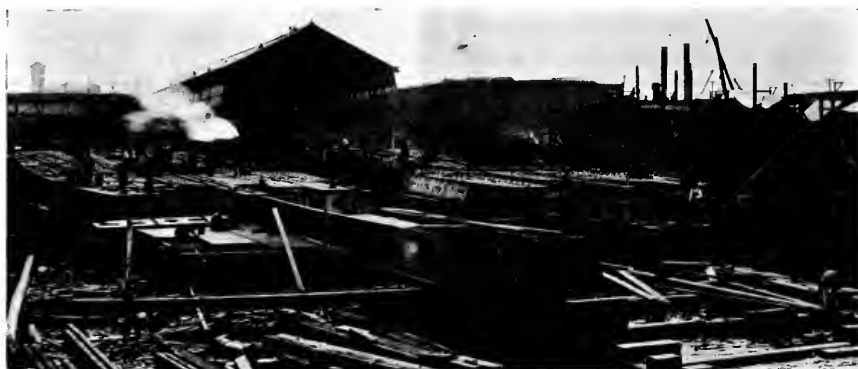
At work on the double bottoms of two new steamers at the yards of the Seattle Construction and Dry Dock Company.
